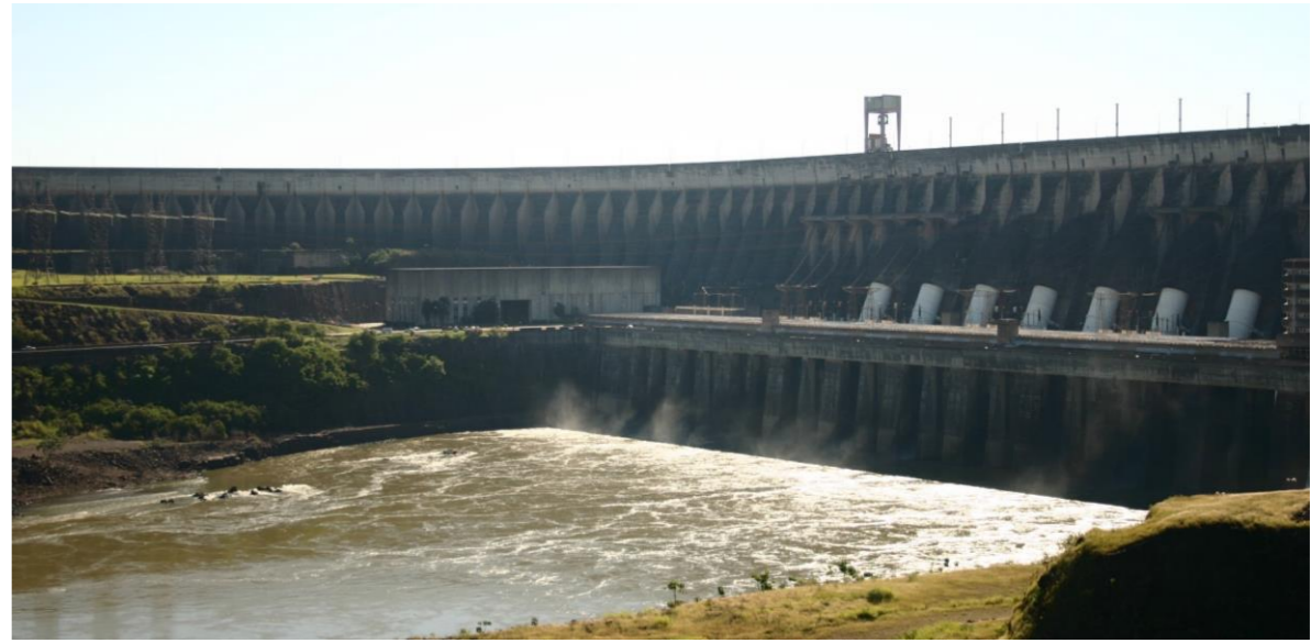
An example hydro power plant Itaipu [1]
