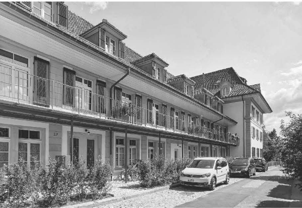
Renovation of Weissensteingut
