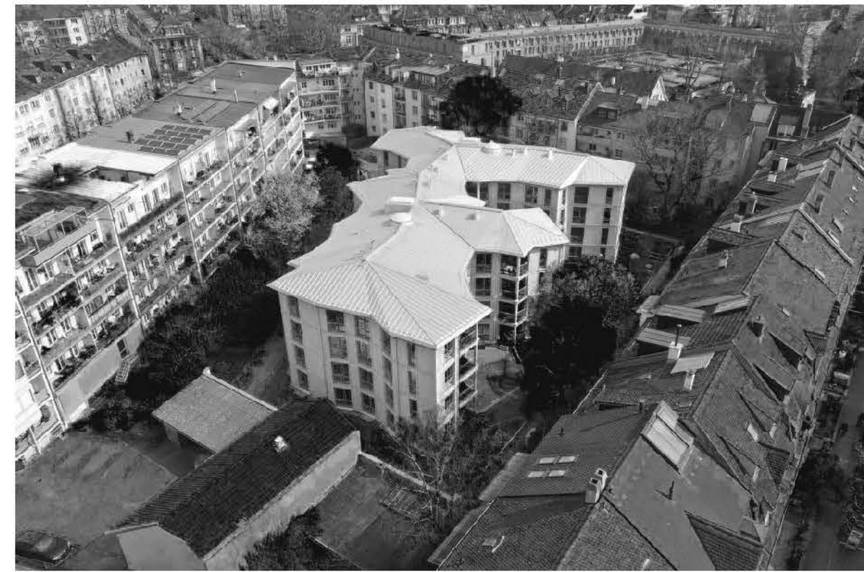
Courtyard Development Riehenring
