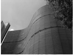
Fig.23. Edifício Copan, photograph from the street
