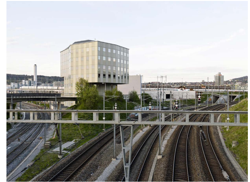
Fig.14. Canteen and offices
