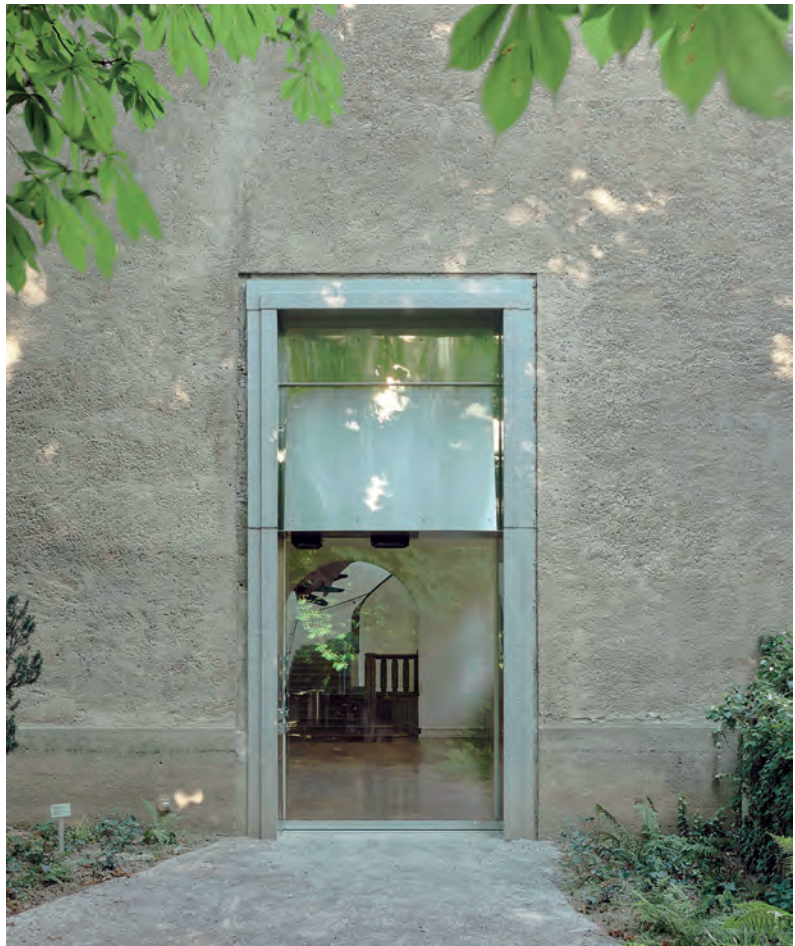
Fig.54 An opening in the wall, no big structural change, yet a big impact.
