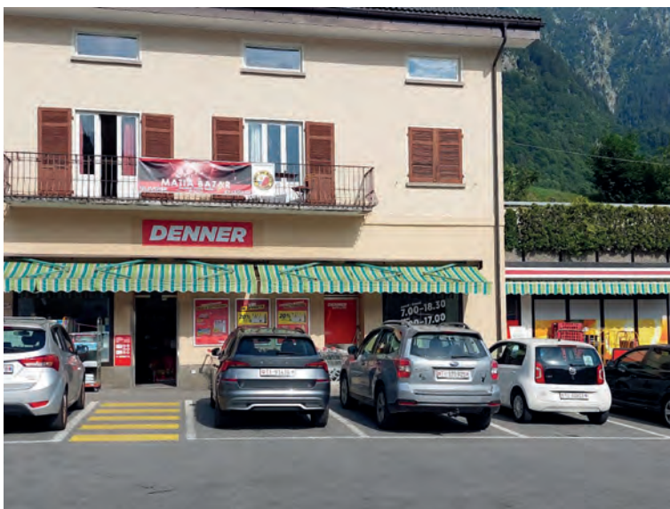
Fig.28 Piazza d'Armi, view to the entrance of Denner, the supermarket
