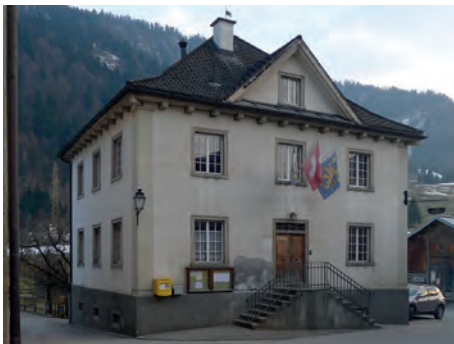
Fig.39 The school building
