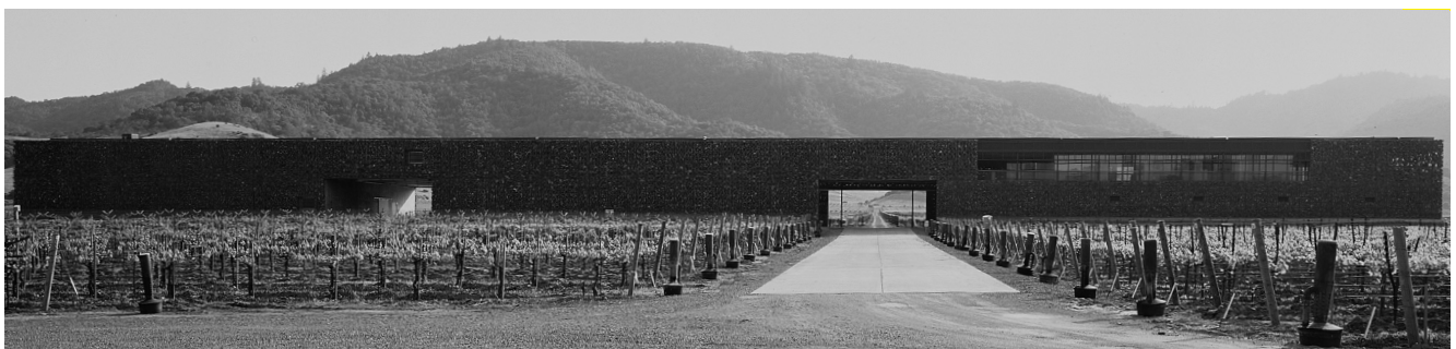
Abb. 15. See-through facade from stacked stones in metal framework.
