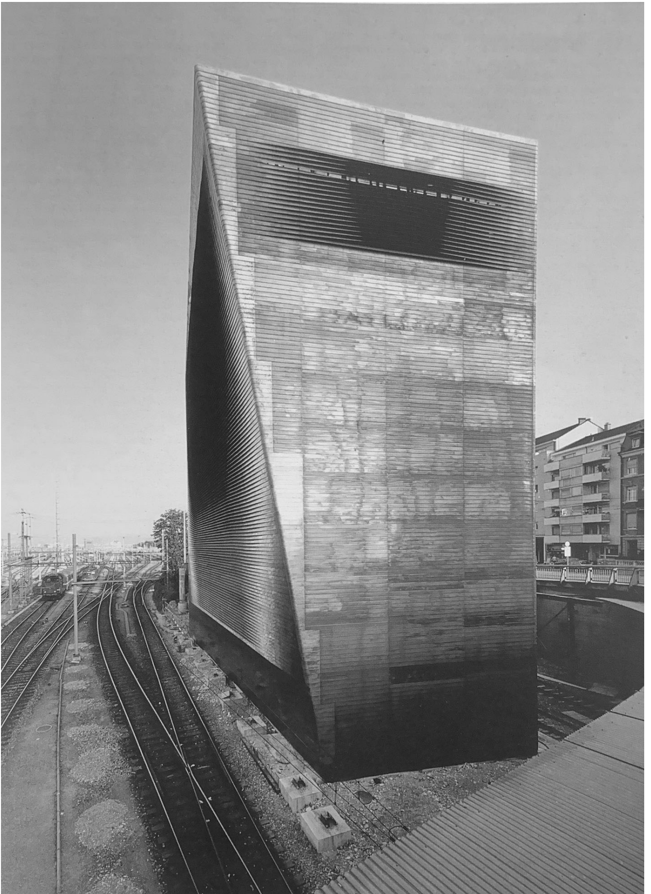
Abb. 33. Copper wrap reminiscing the textile veil. Smoothing edge, unifying the rigid concrete floor steps.
