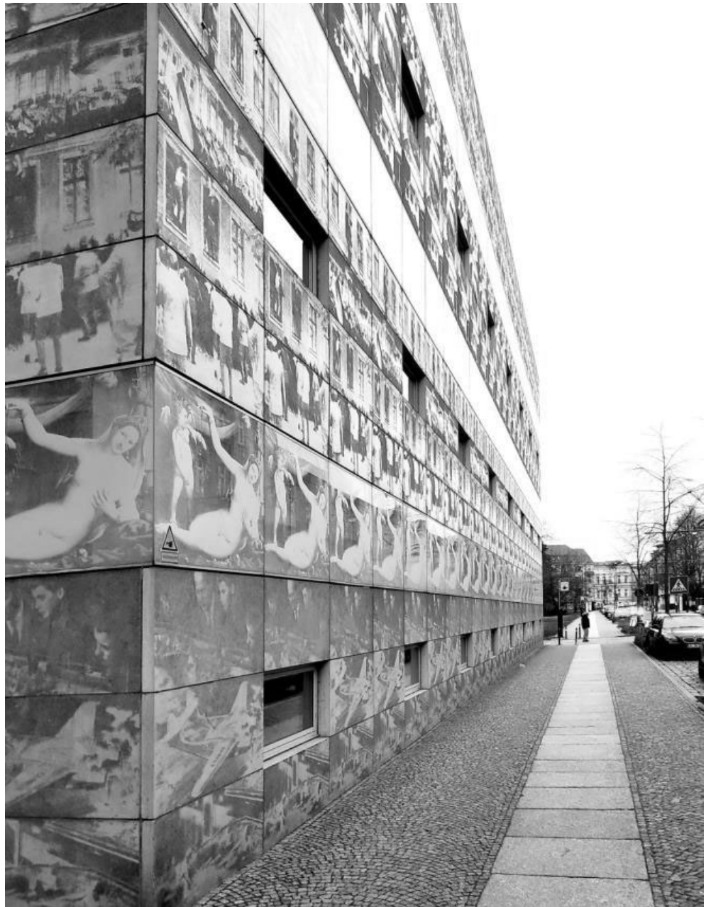
Abb. 35. Rows of imprinted images on glass and concrete with the breaks of windows.
