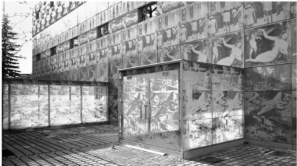
Abb. 37. Visual wrap of the entrances, performed on glass modules. Translucency is emphasized by inner light.
