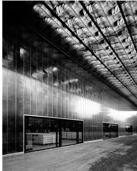
Abb.43. Glimmering light, reflected on semi-matt polycarbonate. Translucency of the roof panels with the same imprints.
