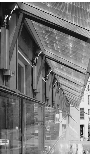
Fig. 31. Open panels at the Suva Haus
