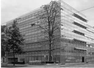
Fig. 15. Suva Haus building after the renovation
