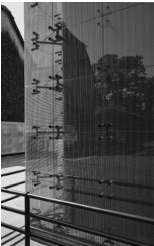
Fig. 42. Steel struts behind the glass skin
