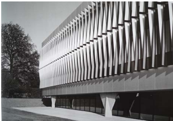
Fig.CS 1: Institute for pathology and forensic medicine, county hospital, St. Gallen. Fixed louvers were calculated and designed to reduce mechanism complexity. This solution reduces maintenance and disturbance.[10]
