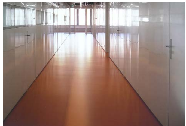
Fig.CS 2: Institute of Pathology and Forensic Medicine, County Hospital, St. Gallen. A PU floor was chosen because it allowed an easy and quick refurbishment, reducing disturbance and increasing acceptance [10]
