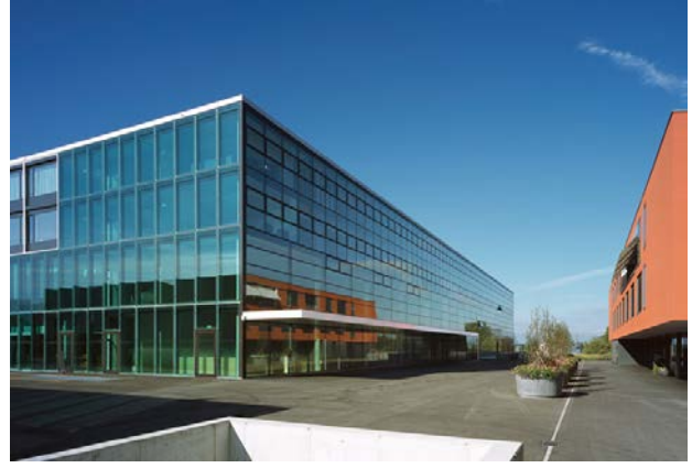
Fig.CS 4: Cantonal Hospital Zug and Care Centre. By constructing the facilities next to each other, high synergies are achieved through sharing services, staff, and underground mechanical engineering [13]
