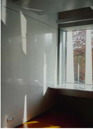
Fig.CS 3: Institute of Pathology and Forensic Medicine, County Hospital, St. Gallen. Metal partition walls can be repositioned and recycled. The reflexion of light contributes to optimal distribution of illumination [10]
