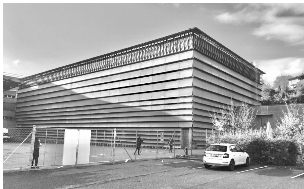
Fig. 8. Ricola Storage in Laufen. View from the arrival area.
