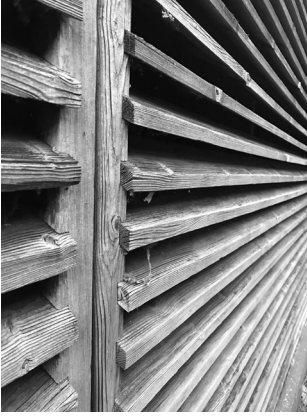
Fig. 13. Wooden fence-like surface of the Shelter in Chur.
