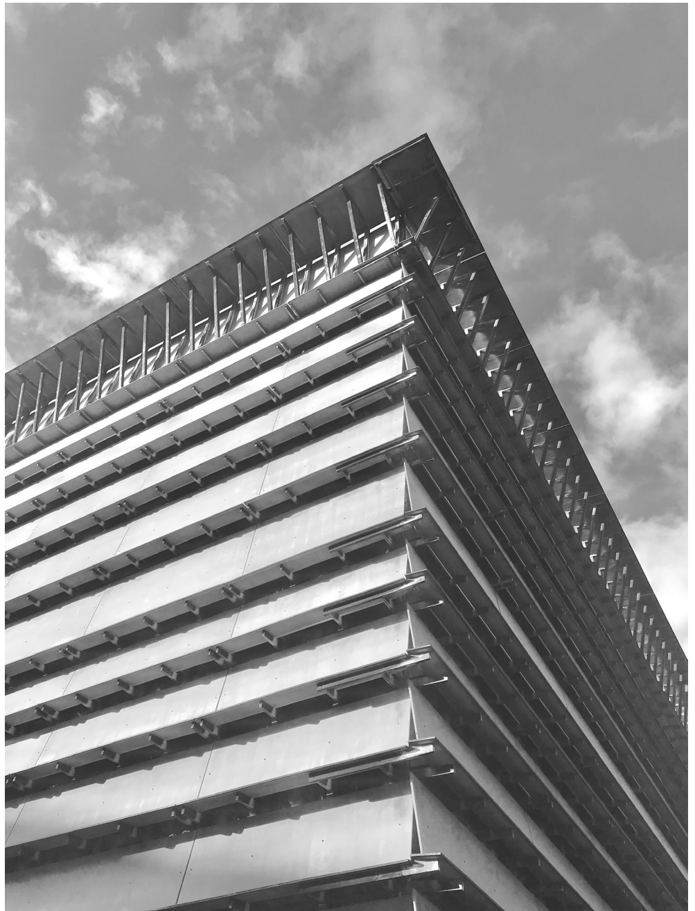
Fig. 11. The cladding of the Ricola Storage Building.
