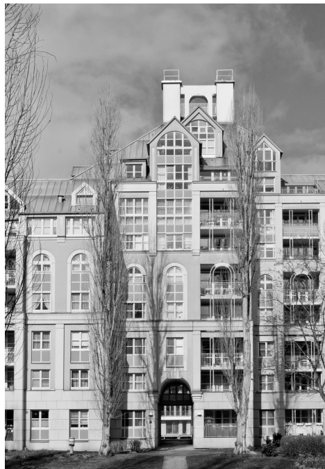
Abb. 13. Housing elevation rising like a mountain
