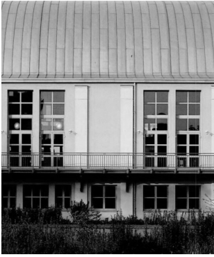
Abb. 18. Humboldt library with classical facade and zinc roof
