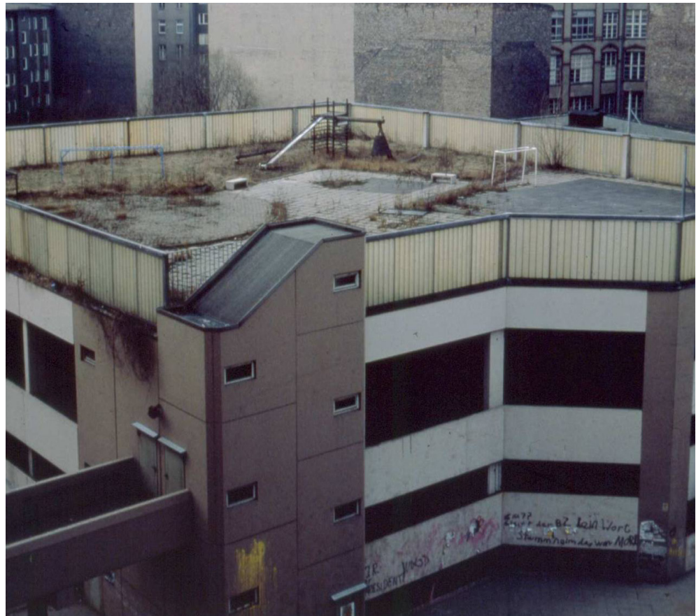
Fig. 14. Parking house in Dresdener Strasse before its transformation.
