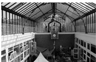
Fig. 17. Photograph of the glasshouse courtyard.
