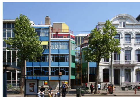
Abb. 32. The colourful new part establishes a relation with the old part of the Hubertus House.
