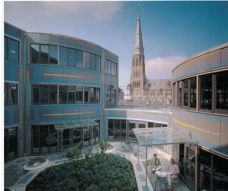
Abb. 43. Terrace garden surrounded by offices on the 2nd floor of Court of Audit.
