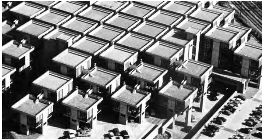
Fig. 01 birds view of the building 1970s
