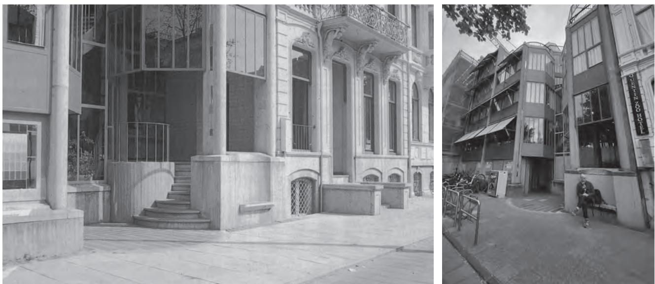
Fig. 23. Entrance looping through the old and new parts of Hubertus house. Fig. 24. The in-between realm.
