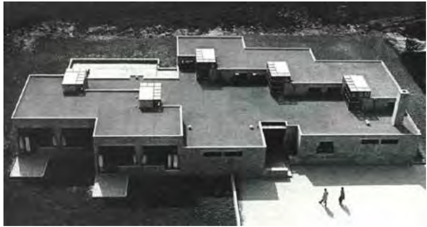
Aerial view of the building after the first two construction phases were finished.
