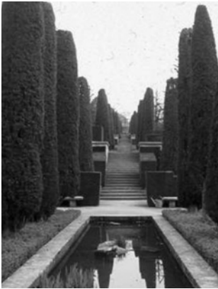
Fig. 23. Cemetery of Bois du Vaux by A. Laverrière in Lausanne, 1926
