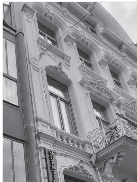
Fig. 33. The window frames of the old building are coloured to indicate a relation between old and new.
