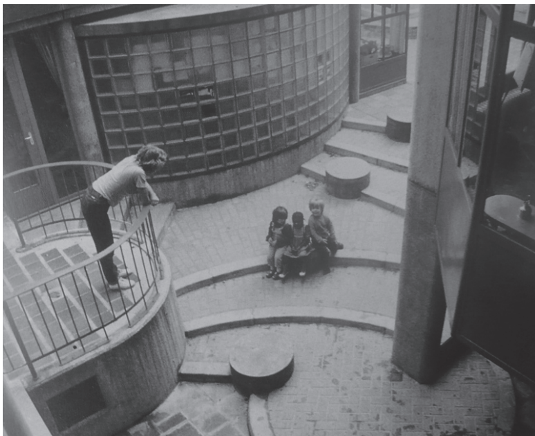
Fig. 42. Windows of the canteen.
