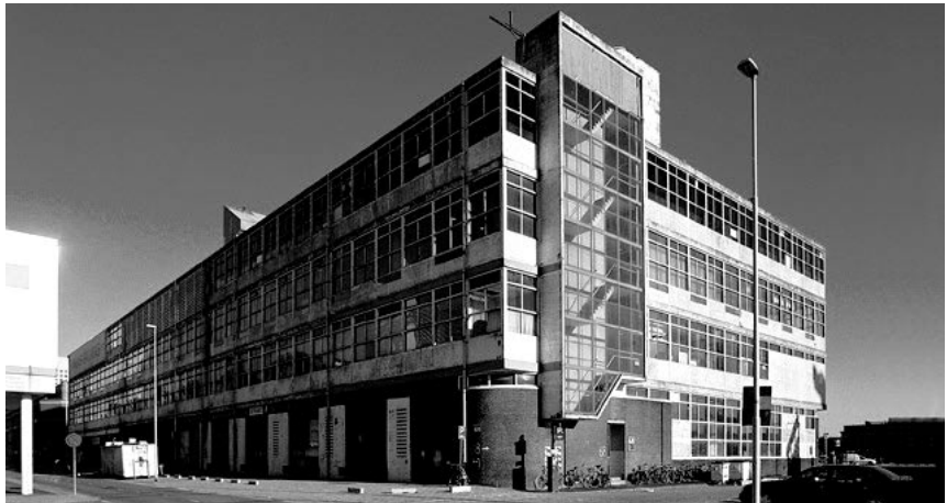
street view before renovation
