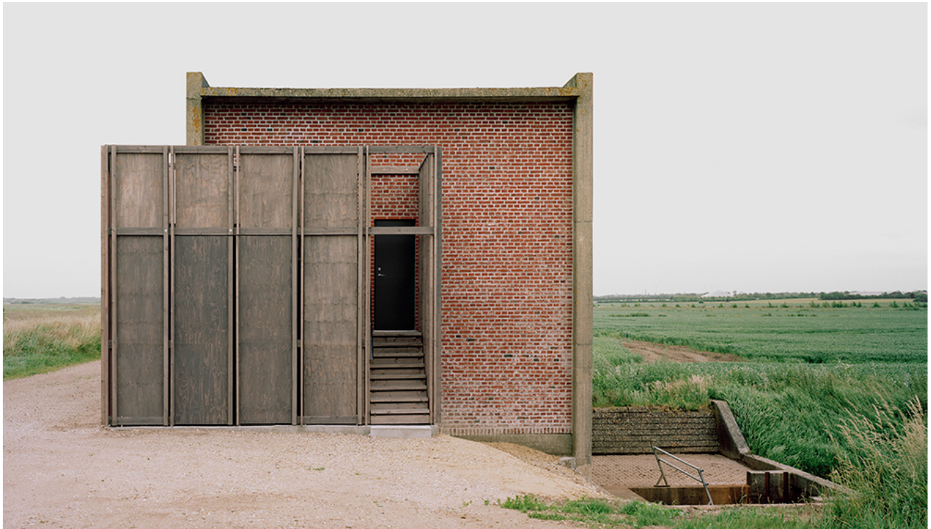
Johansen Skovsted, Pump Station South. Photo: Rasmus Norlander
