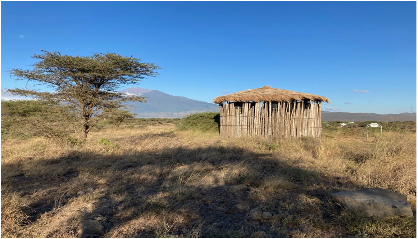
Current water infrastructure on the school campus, Mount Kilimanjaro in the background (photo: Gunter Klix)
