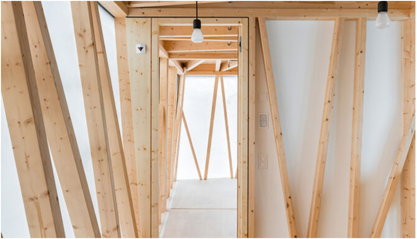
NFS Digitale Fabrikation, Spatial Timber Assemblies, DFAB House, NEST in Dübendorf. (Photo: Roman Keller)
